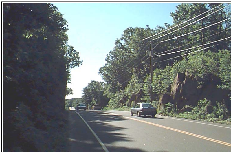
View of Route 64 with limited sight distance and rock ledge on both sides of the roadway
