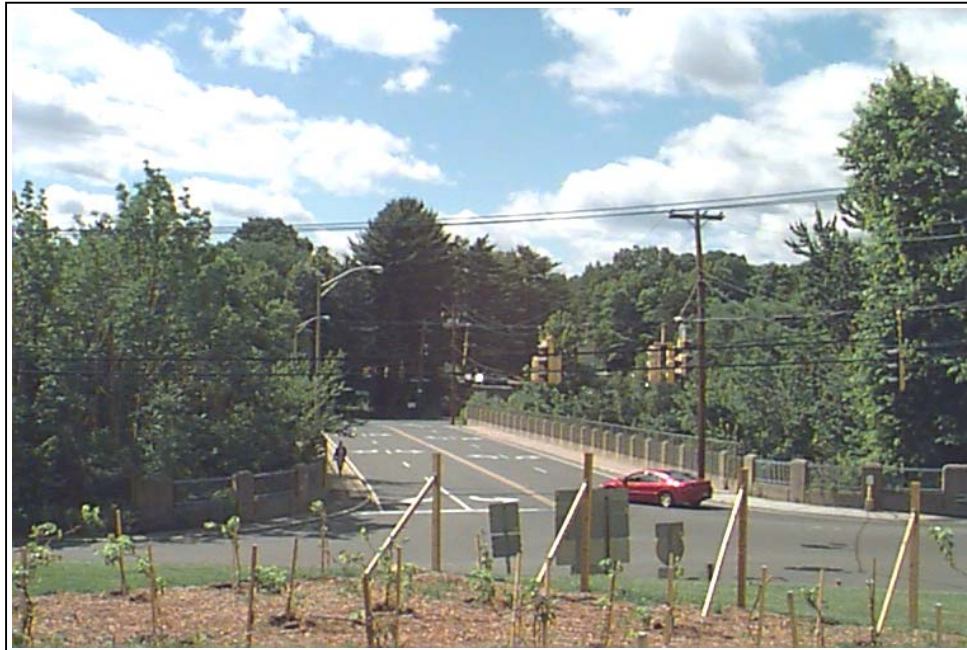
View of the Chase Parkway bridge over I-84
